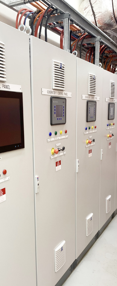
Photo: New Generator Control and SCADA System for 12MW of back up power across 7 No. New and existing engines.
